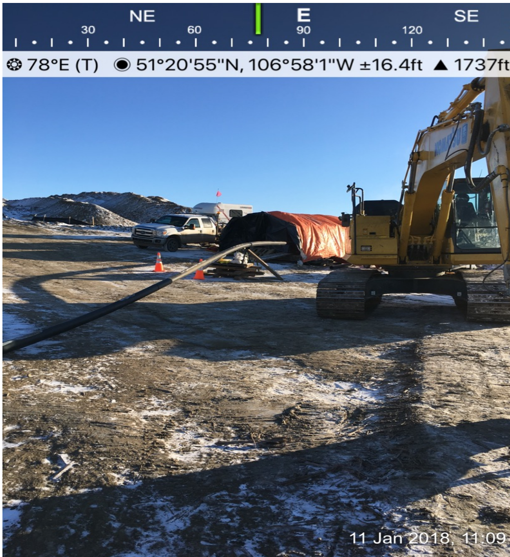
INFUSING BUOYANCY LINE INTO BORE SECTION
