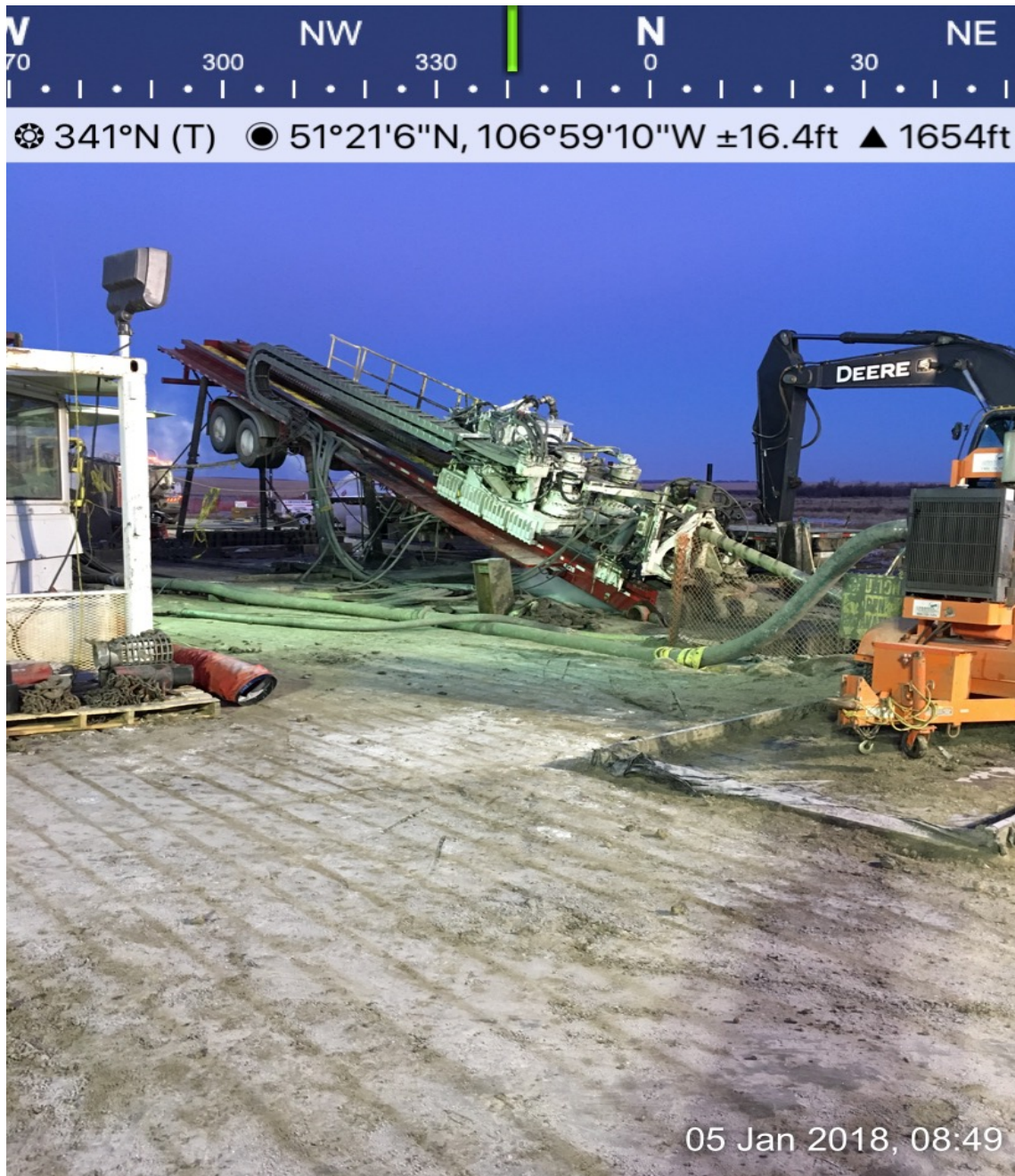
ENTRY POINT OF HORIZONTAL DIRECTIONAL DRILLING
