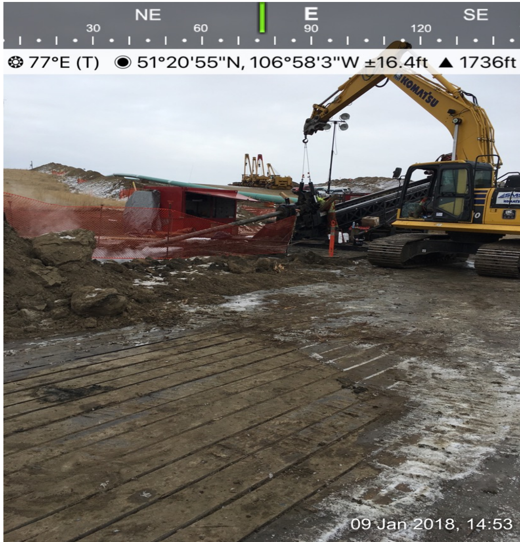
Exit point of Horizontal Directional Drilling
