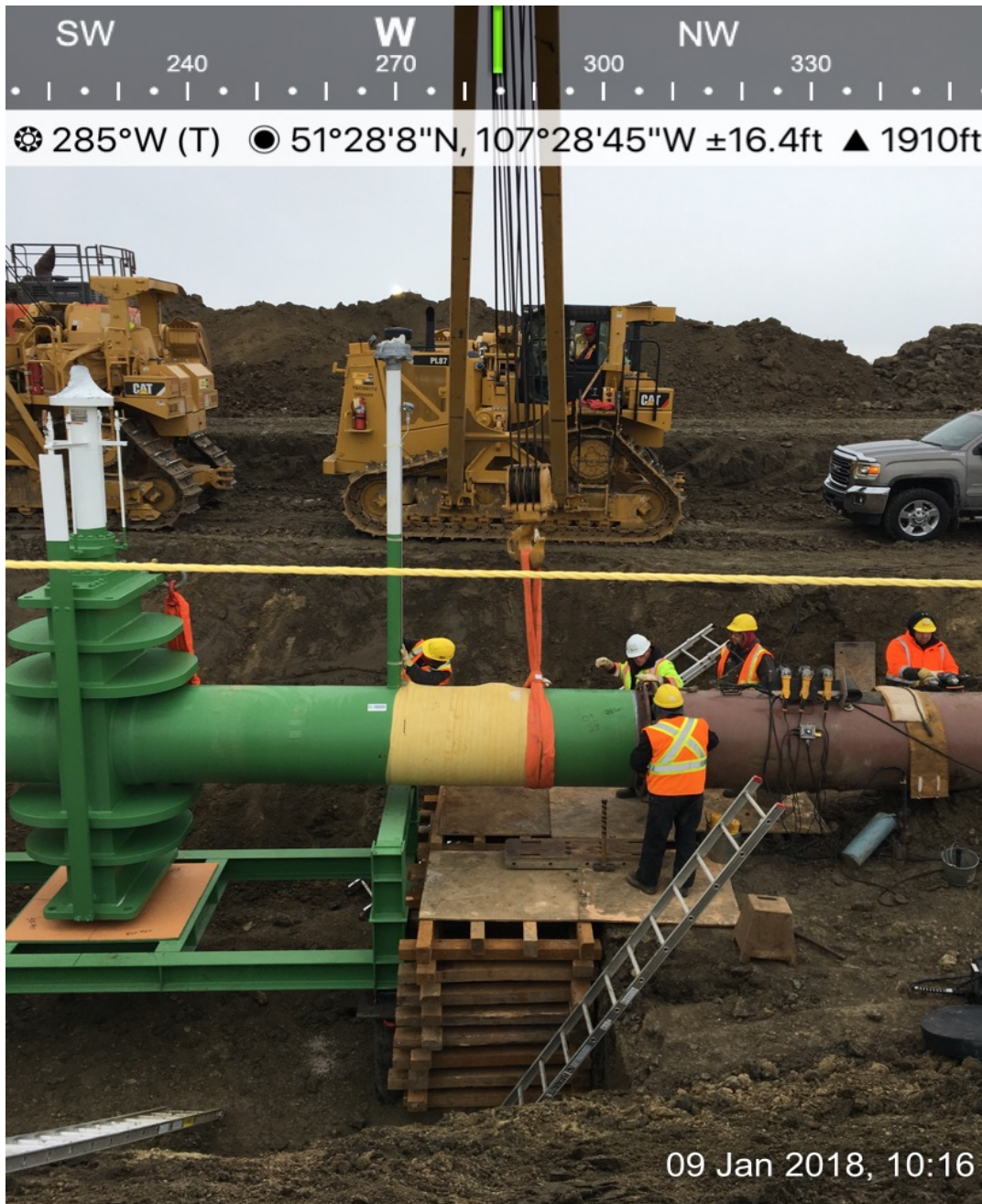
VALVEINSTALLATION
