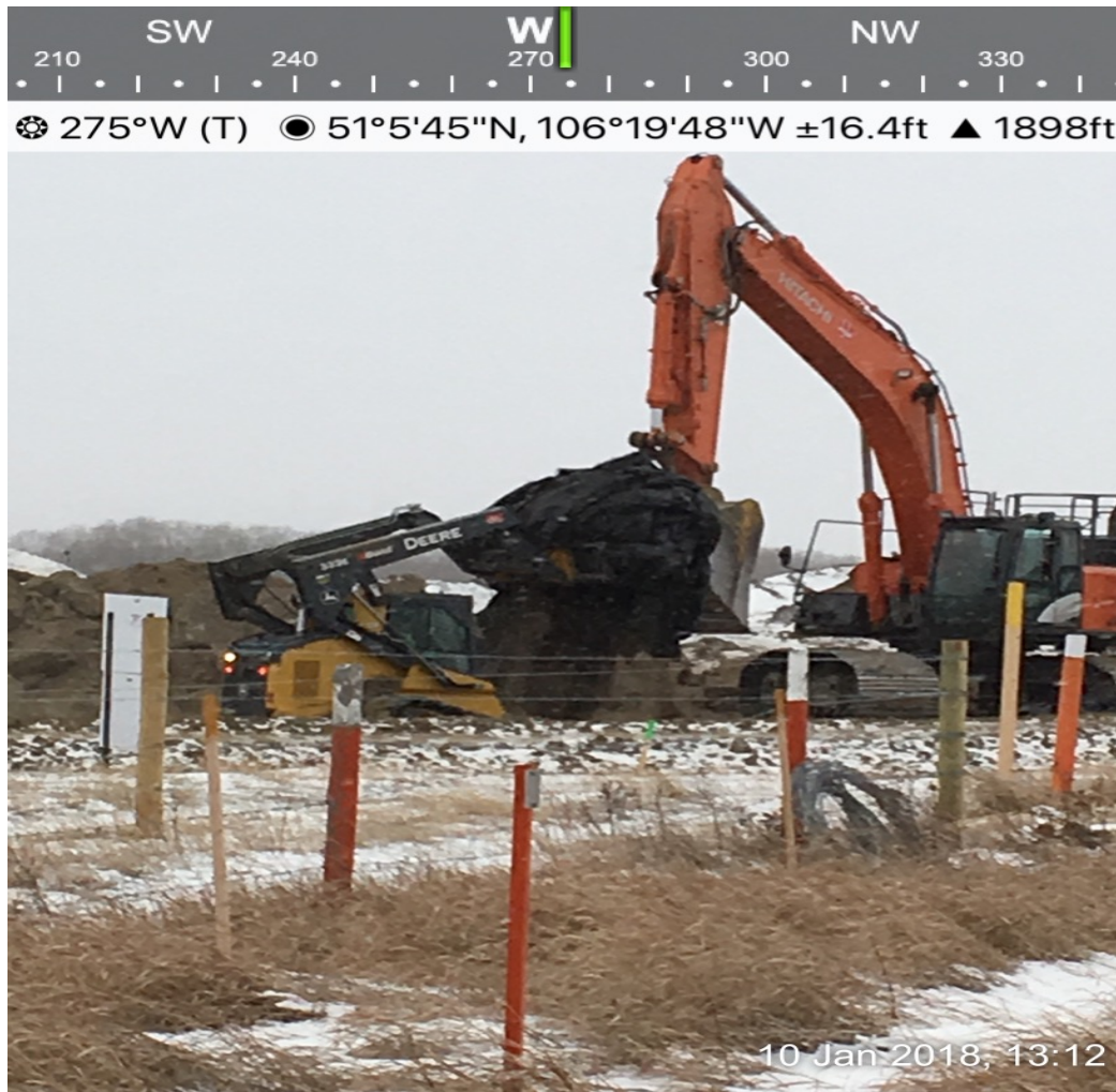
Removing Geotech material from access approach
