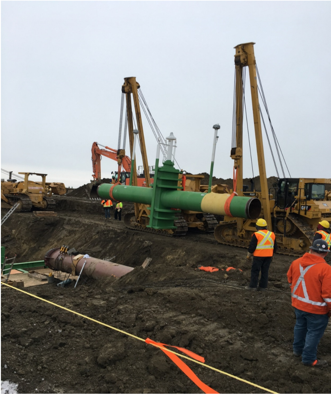
INSTALLATION OF VALVE
