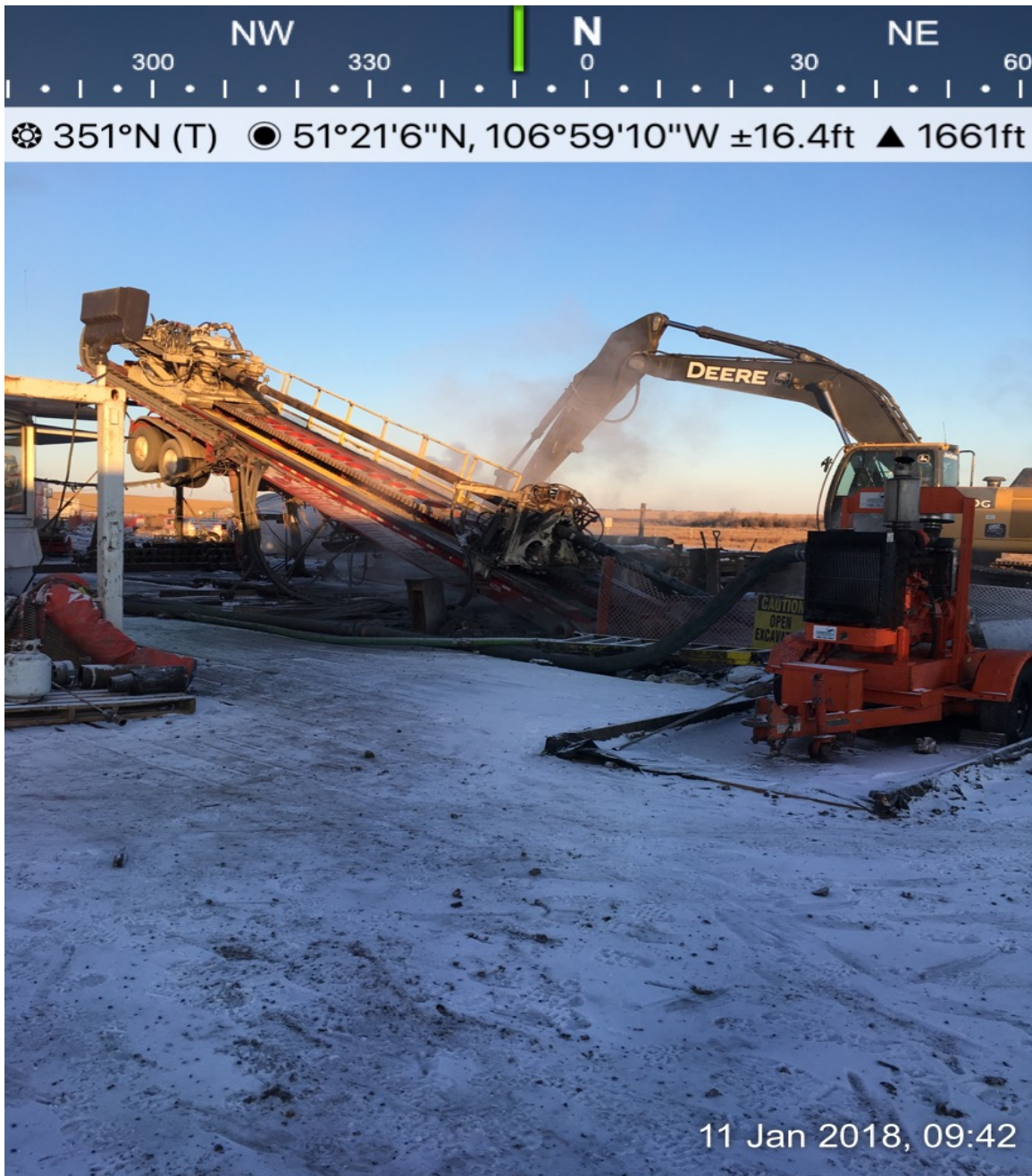
ENTRY POINT OF HORIZONTAL DIRECTIONAL DRILLING
